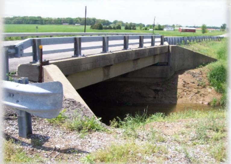
The concrete bridge over Lakey's Creek.
