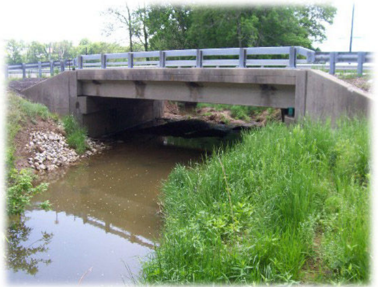
A view of Lakey's Creek as it travels under the bridge.
