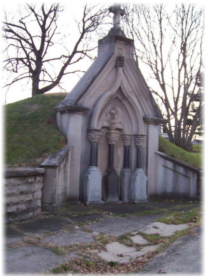
This crypt has been sealed, and is rumored to lead into the underground tunnels.
