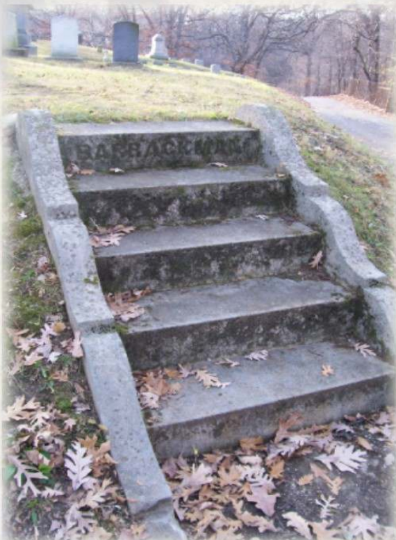
The Barrackman Staircase.
