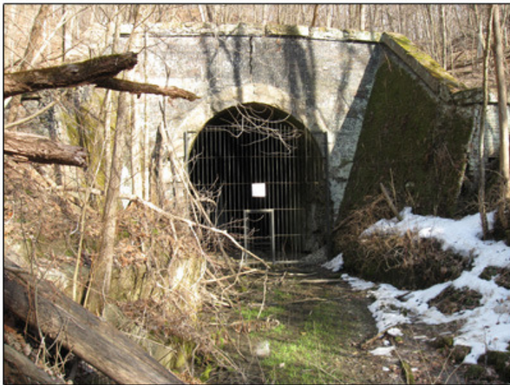
Nature slowly reclaims the Winston Tunnel.
