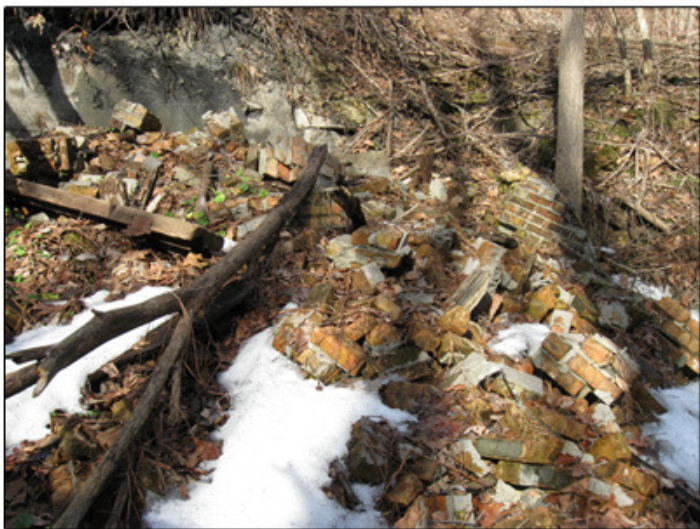
A pile of bricks is all that remains of the former pump house, which was torn down in 2007.
