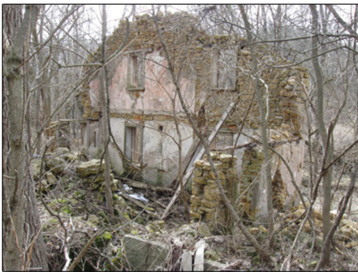
The ruins of a stately brick and plaster home sit near the trail leading to the Winston Tunnel.
